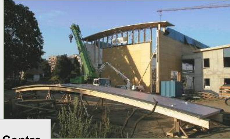
inverted bowstring CLT element
