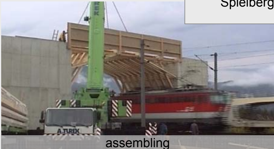
carriageway slab: 19-layered CLT element
