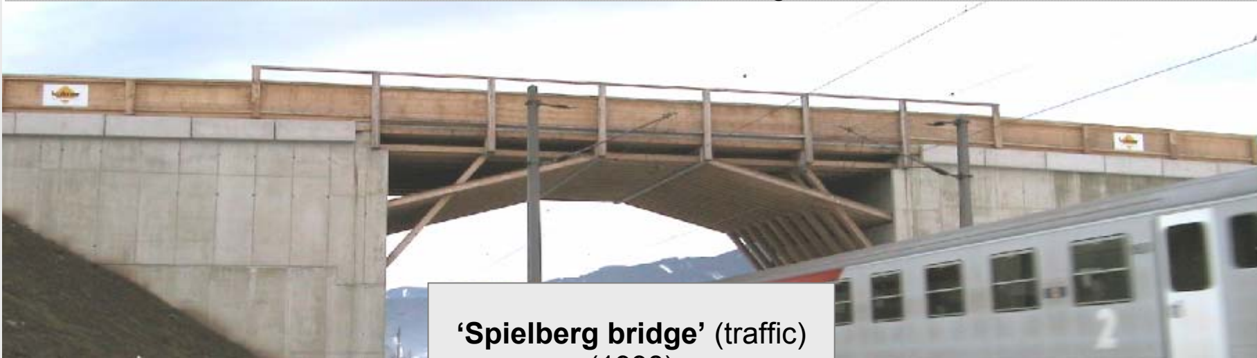
view of the finished bridge
